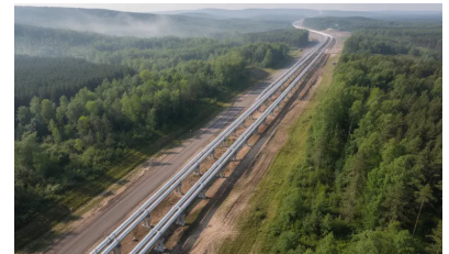
Natural gas infrastructure. Illustrative photograph.
